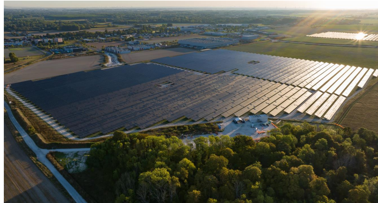
The Romilly 42.7-MWp solar farm with 80,000 solar panels - Equans
