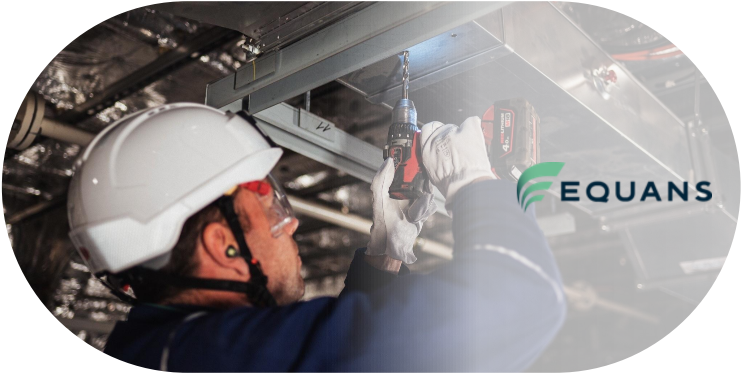
Axima Marine (Equans) is equipping Multi-Mission frigates with an HVAC and NRBC (Nuclear, Radiological, Biological and Chemical) protection system
