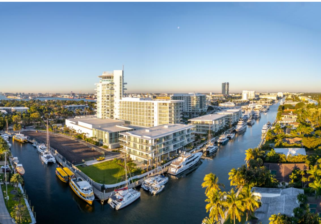
Renovation of the Pier Sixty-Six tower in Fort Lauderdale, Florida (Bouygues Construction)
