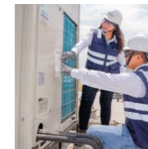
Equans Rechenzentrum in Peru
