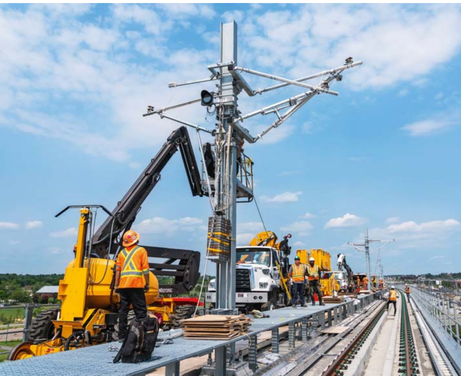
Installation of the brackets used to attach the catenary wires to the poles.
