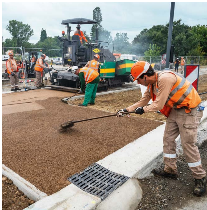
↶ Workers pass the finisher over just-laid asphalt.
