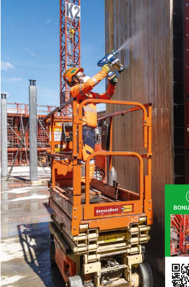
← Applying formwork oil with a pulveriser.
