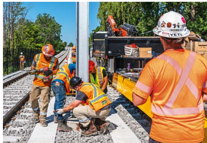
Installation of the brackets used to attach the catenary wires to the poles.
