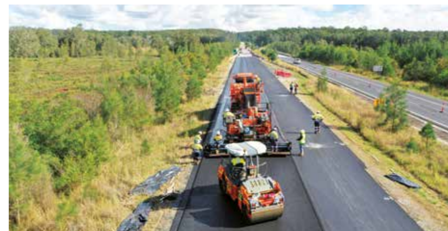
AUSTRALIA – A Colas Australia team lays SMA10-graded asphalt on a road near Clybucca, New South Wales.
