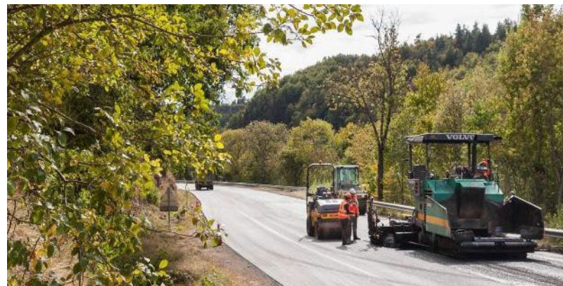
Applying a cold asphalt mix to a road - France
