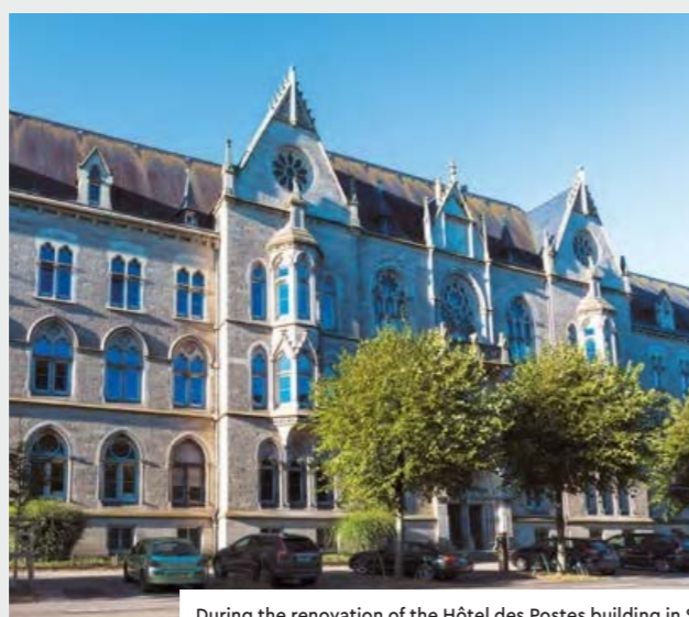
During the renovation of the Hôtel des Postes building in Strasbourg, 20,000 m 2 of existing structure was kept, 1,000 wooden window frames repurposed and 2,700 m 2 of carpet recycled.
