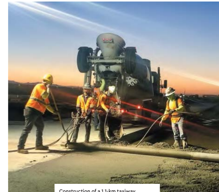
Construction of a 1.1-km taxiway at Los Angeles international airport
