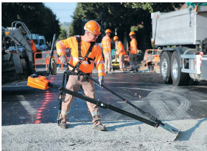
The ExoPush exoskeleton, presented at Vivattech 2018, reduces the physical effort of spreading asphalt while improving working conditions.
