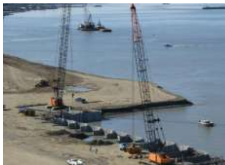
Extension of the port of Anchorage, Alaska
