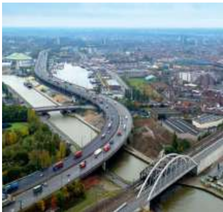
Refurbishment of the Antwerp ring road, Belgium
