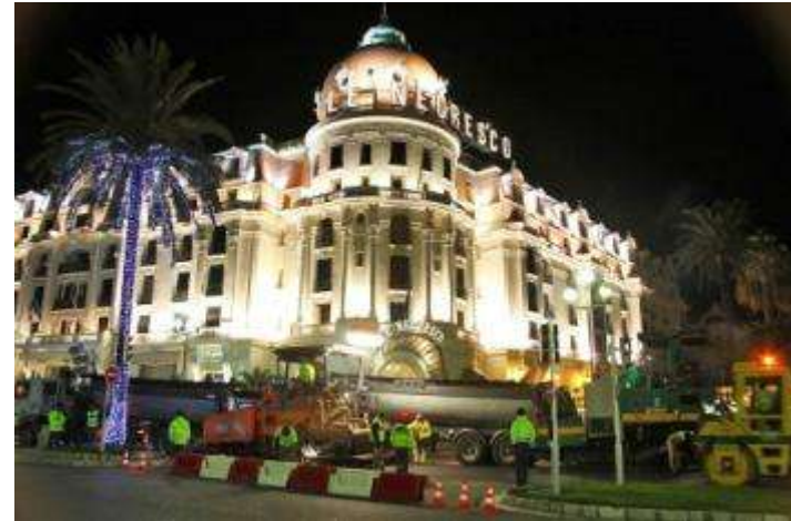
Works on the “Promenade des Anglais” in Nice, France
