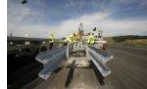
Road safety works
