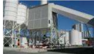
Ready mix concrete plants
