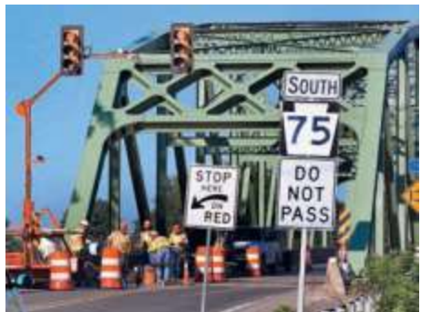
Refurbishing a bridge in Port Royal, Pennsylvania
