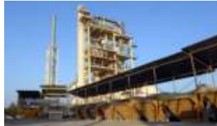
Asphalt mixing plants
