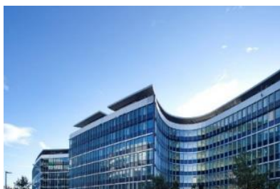
Green Office ® Rueil, head office of Unilever France
