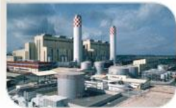
Lagos thermal power plant
