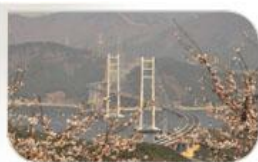
Masan Bay Bridge, South Korea
