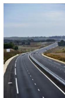
The A75 motorway, Southern France
