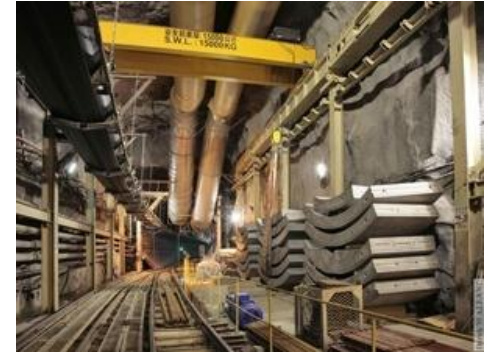
Tunnel, Hong Kong
