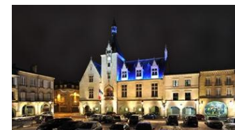
Public lighting, Libourne
