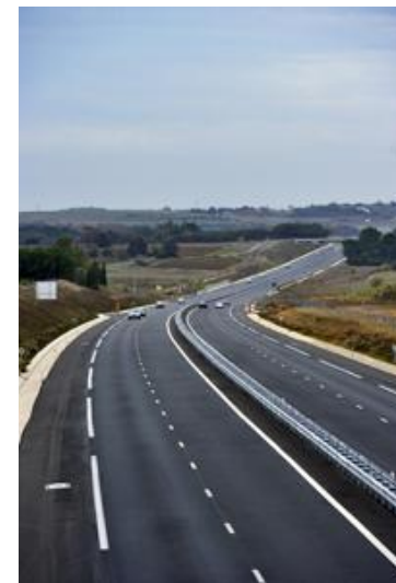
The A75 motorway, Southern France
