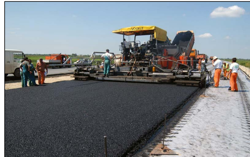
Application of asphalt mix, Hungary
