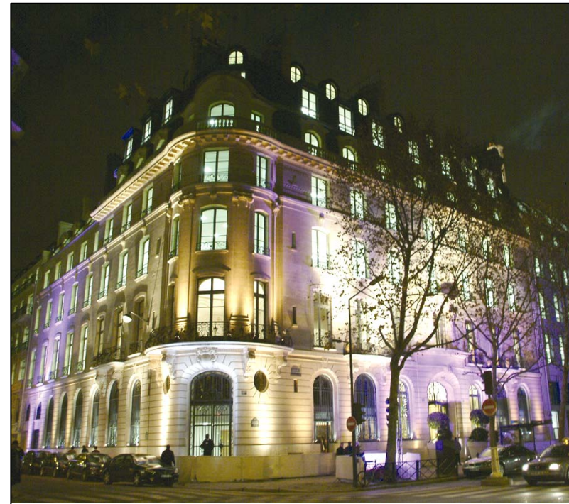
96 boulevard Haussmann, Paris Renovation of former Indosuez head office
