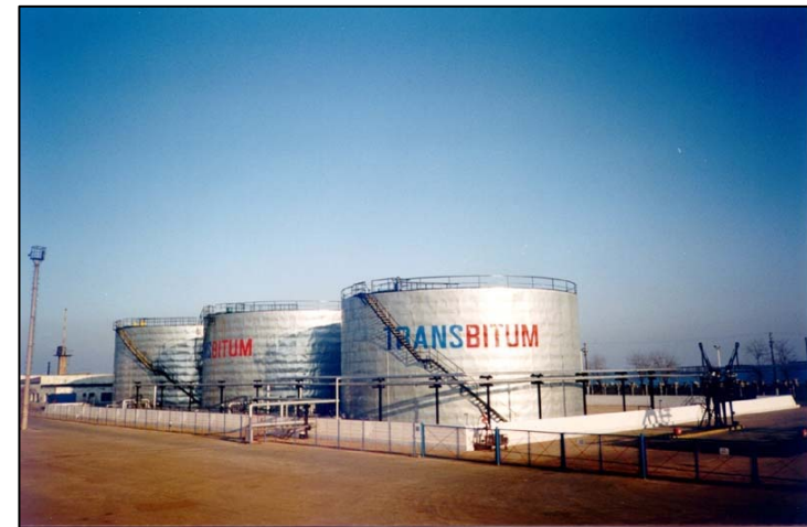
Transbitum storage plant Mangalia port, Romania
