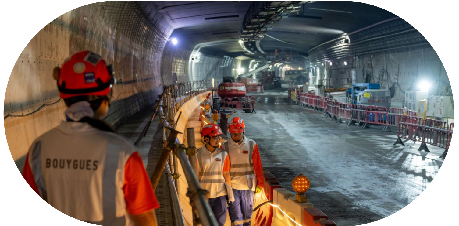
Trunk Road T2 subsea road tunnel in Hong Kong – Bouygues Construction
