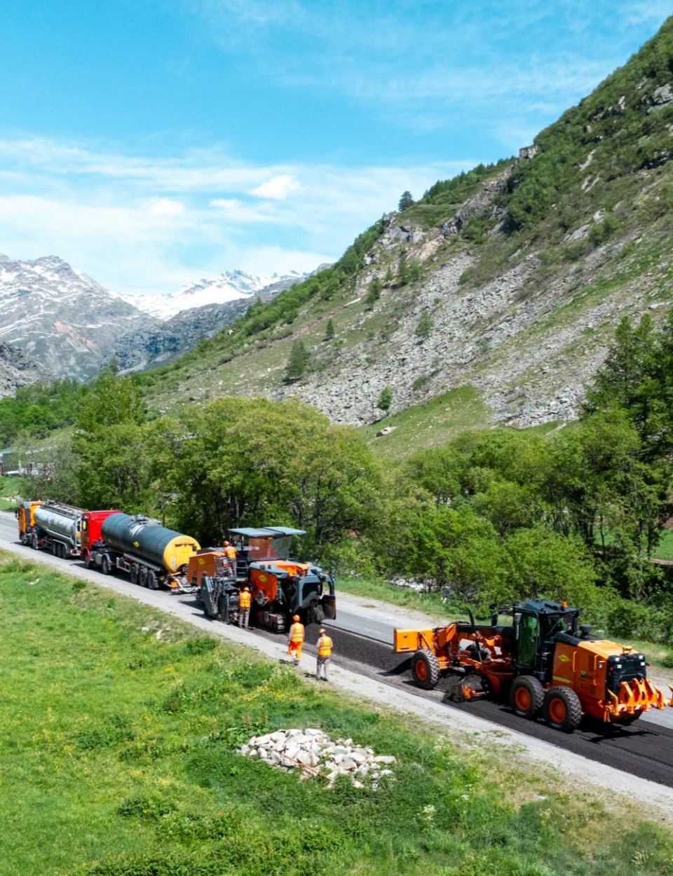
Laying of Recycol in the French Alps – Colas
