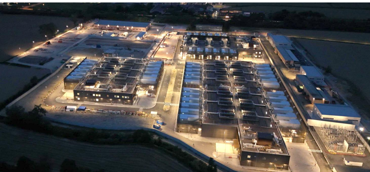
MIL04 data centre project in Italy - Equans
