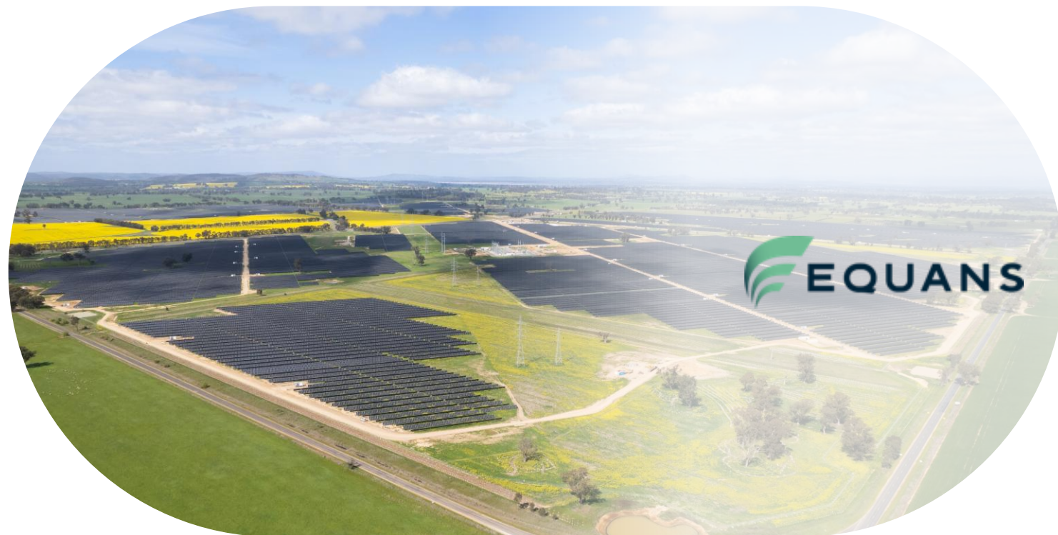
Goorambat solar farm in Australia – Equans
