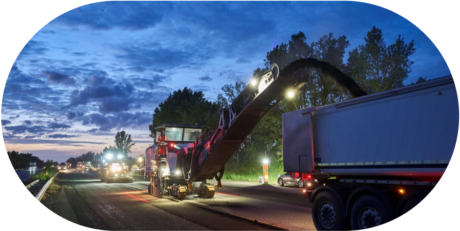
Aximum (Colas) working on the A61 road resurfacing project in Toulouse.
