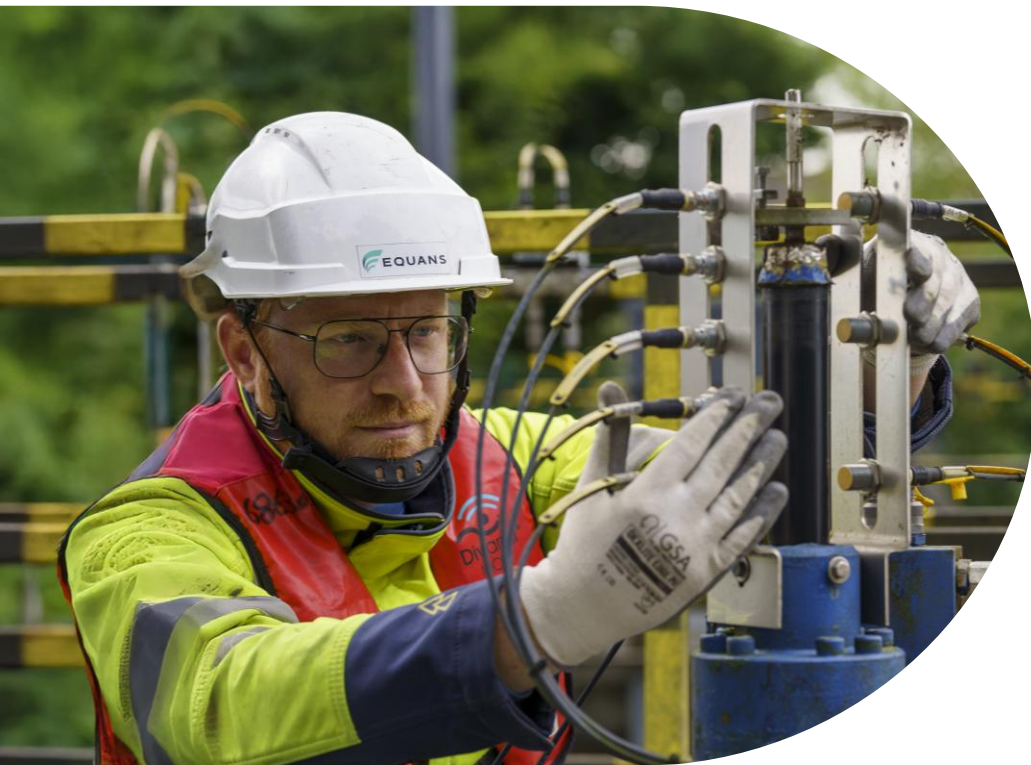
Electro-hydraulic renovation on the Dessel-Turnhout-Schoten canal, Belgium - Equans
