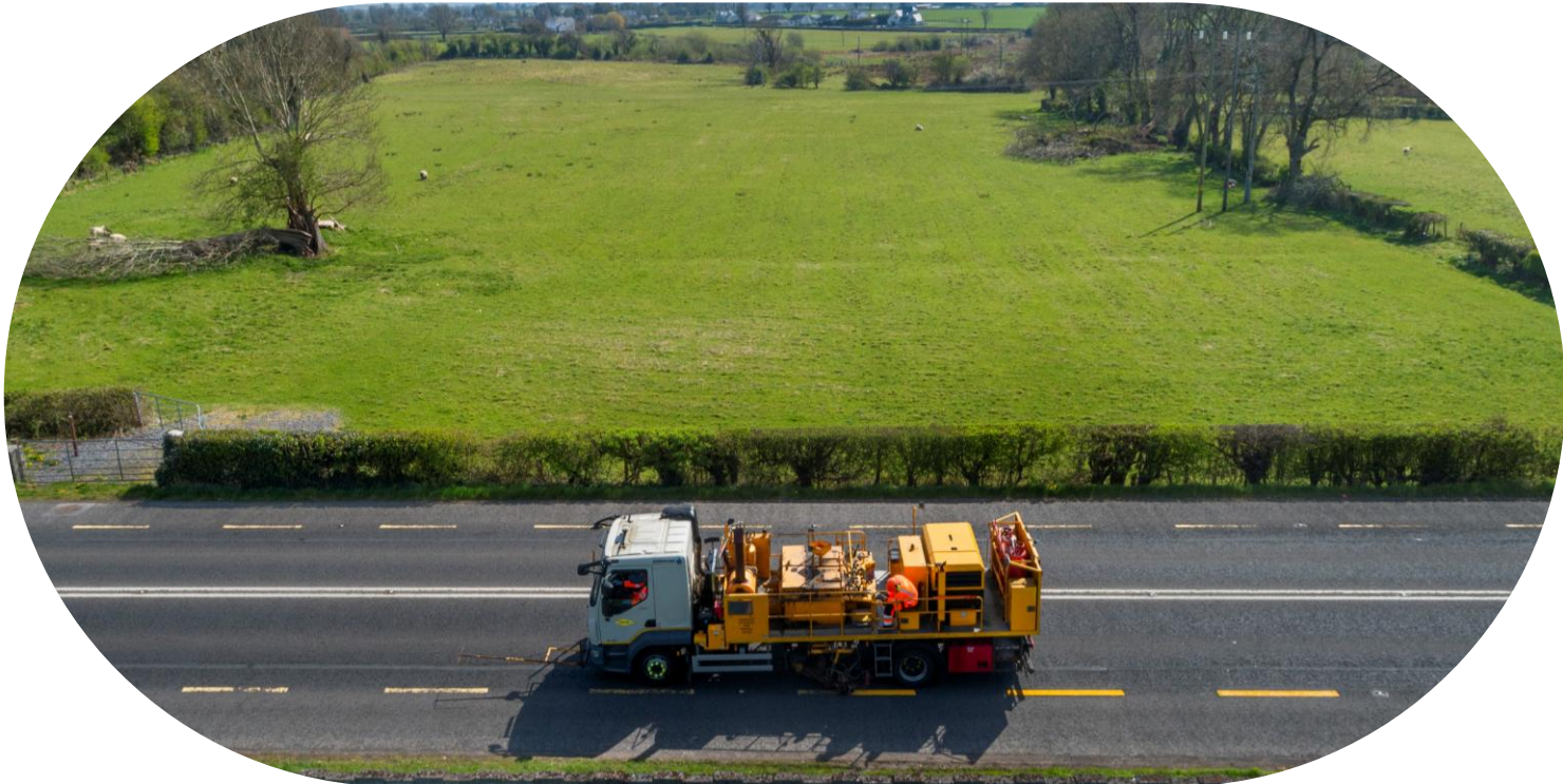
Road marking work on the N63 road in Ireland (Colas Ireland)
