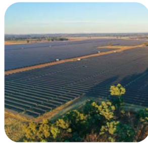
Culcain Solar Farm, a solar project spanning over 1,000 hectares in Australia (Bouygues Construction and Equans)
