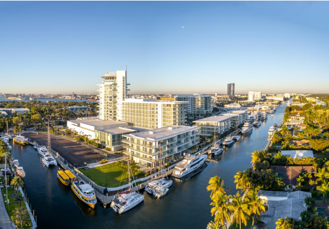
Renovation of the Pier Sixty-Six tower in Fort Lauderdale, Florida, by Bouygues Construction
