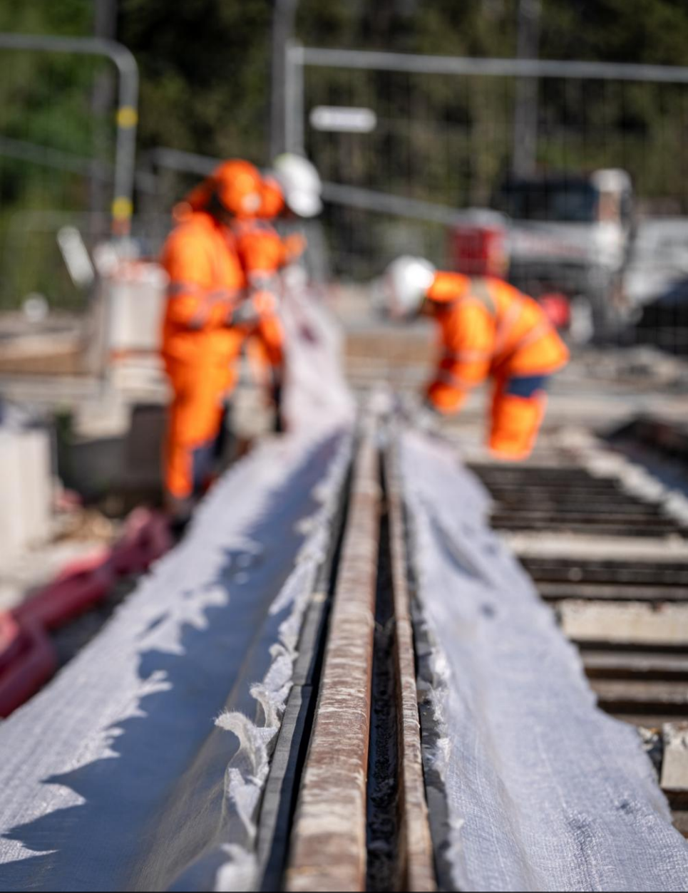
Track laying for Line 5 of the Montpellier tram system (Colas Rail)
