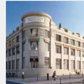
Conversion of the Hôtel des Postes building into a retirement home in Châteauroux, France (Bouygues Immobilier's Converso solution)
