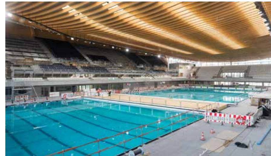
FRANCE – The Saint-Denis Aquatics Centre, built by Bouygues Bâtiment Ile-de-France, has a concave timber frame made up of 90 curved catenary beams, each 55 cm thick and spanning 90 metres. A timber-frame construction record!
