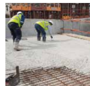
Low-carbon concrete at Bouygues Construction
