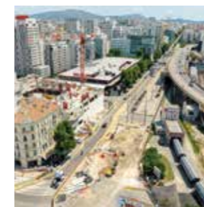
Extension of the T3 tram line in Marseille (Colas)
