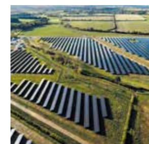
A solar farm in the United Kingdom (Equans Solar and Storage)
