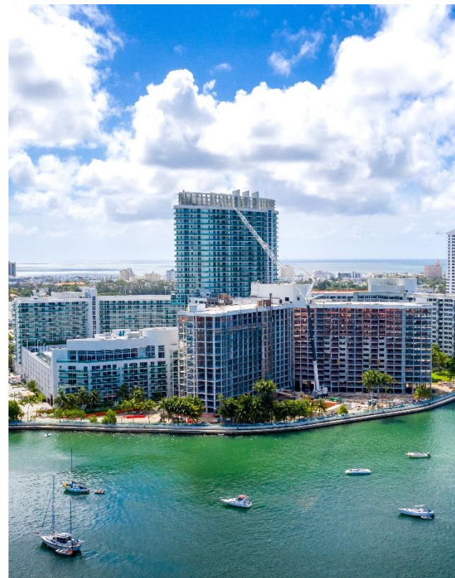
First renovation project in the US – Flamingo Point Center – Miami
