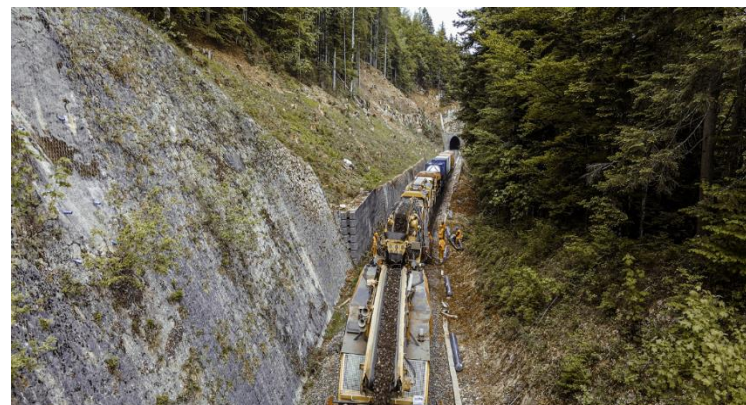
Renewal of the Watchmakers' rails – Eastern France
