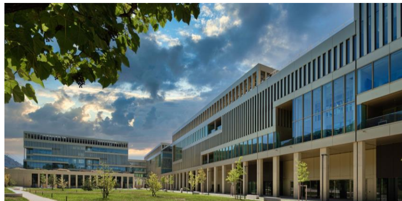
IntenCity - Office building – France (Architect : Groupe 6 – Picture: Creative Buildings)
