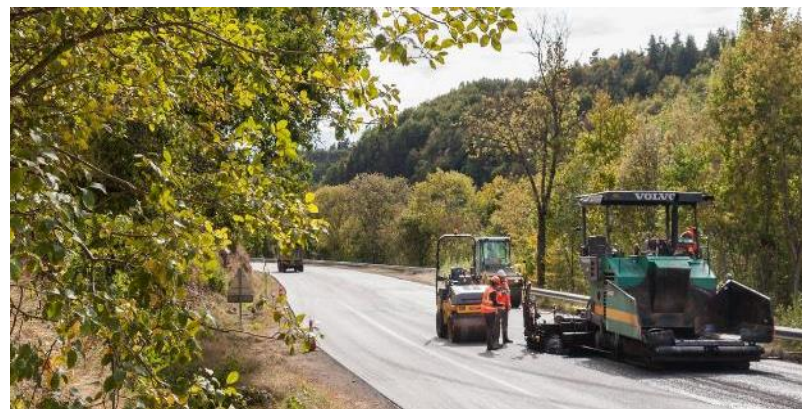
Applying a cold asphalt mix to a road - France
