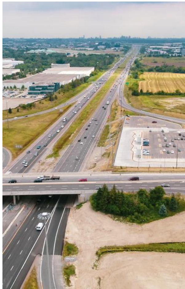
Highway 404 – Ontario – Canada
