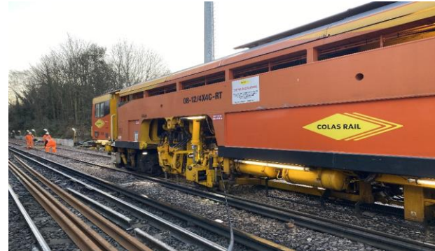
Work on railway lines for Network Rail – United Kingdom
