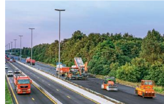
Rehabilitation of 9 km of the E34 motorway: all material recovered from the previous infrastructure was incorporated into the new road pavement
