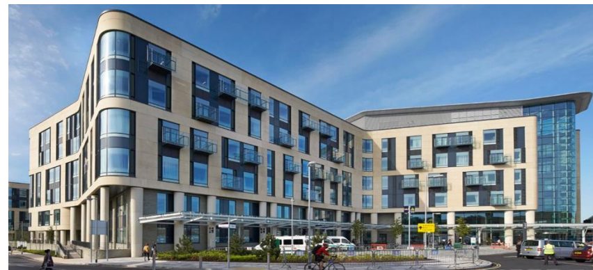
Maintenance at Southmead Hospital – United Kingdom – €159m
