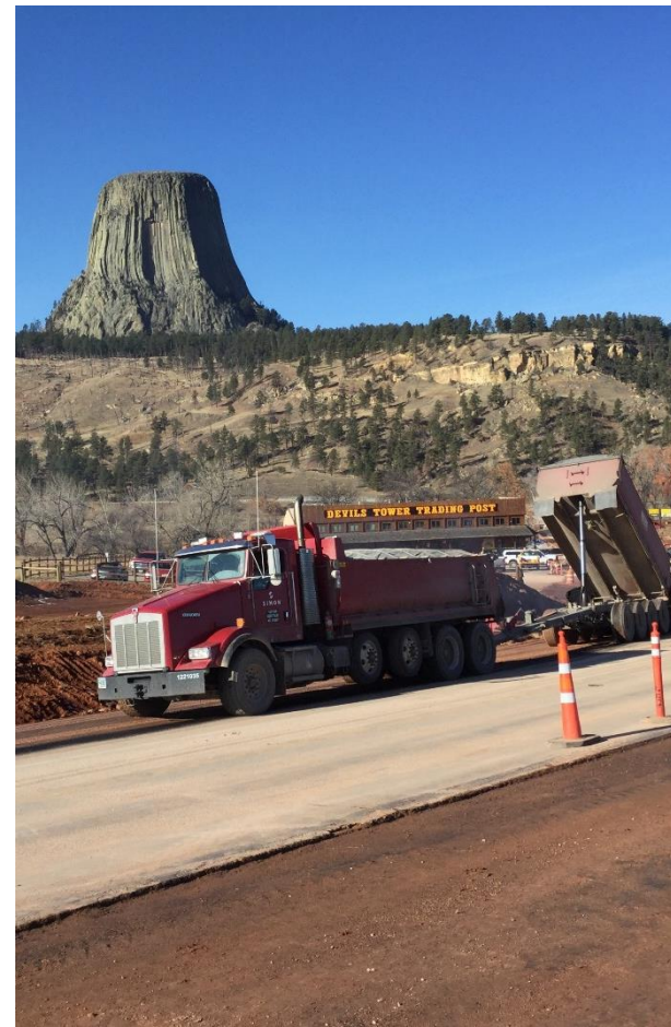
Roadworks at Devils Tower in Wyoming – USA
