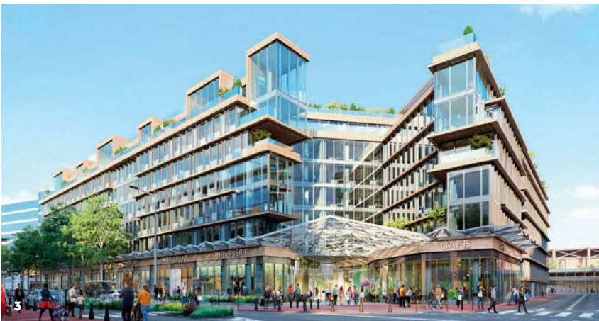
1. Cité Curial-Cambrai in north-east Paris, whose 1,772 housing units were renovated without requiring residents to leave. This was done notably by improving insulation from the outside. 2. Bouygues Construction is renovating the building at 17 boulevard Morland in the centre of Paris. Renovation of the offices at this location is due to be certified by the HQE™ Excellent, BREEAM Bespoke International Very Good and BBC-effinergie® labels. The housing units carry the labels HQE™ Excellent and BBC-effinergie® Rénovation. 3. Sways (Smart Ways to Work), the Rehagreen renovation project to provide flexible office space, in Issy-les-Moulineaux.
