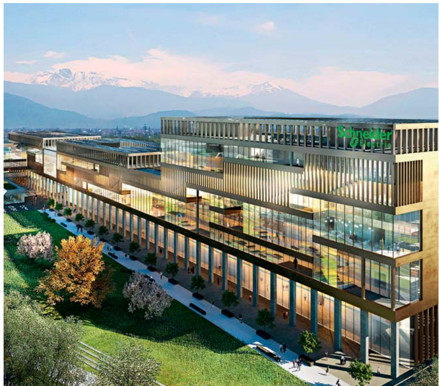
In Grenoble, the future business campus of Schneider Electric will include a 4,000 m 2 photovoltaic power plant, two roof-top wind turbines and a geothermal energy system using groundwater.
