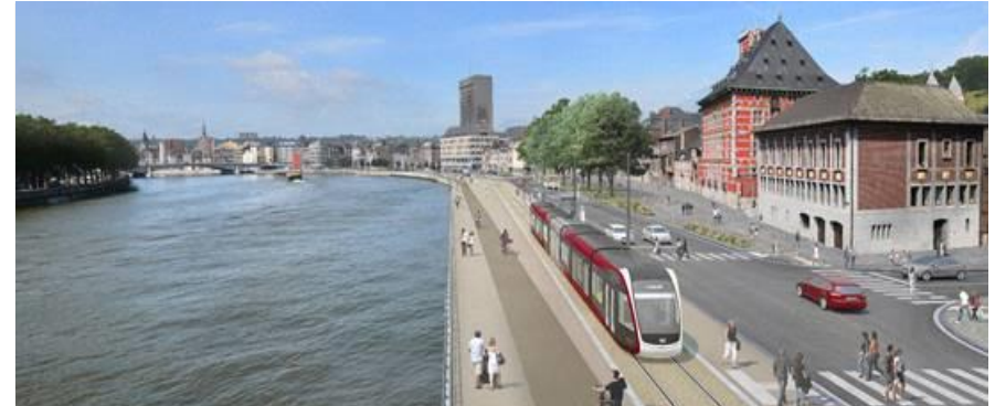
Construction of Liège tram line – Belgium (€266m, excluding maintenance)
