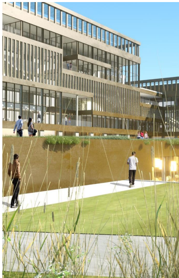
Xpole – Grenoble – France
