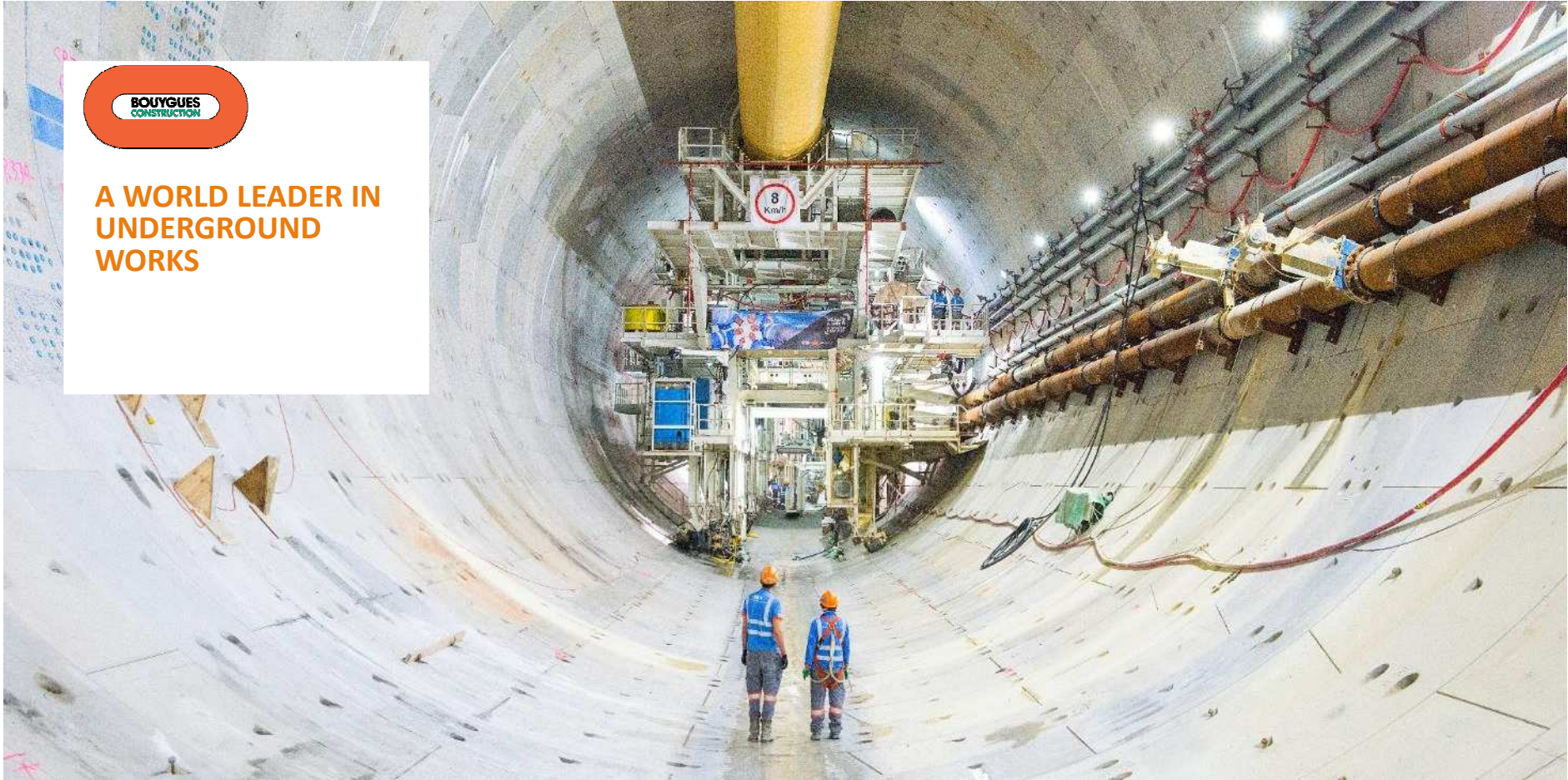
Tuen Mun-Chek Lap Kok tunnel with the world's largest diameter TBM (17.6 meters)
