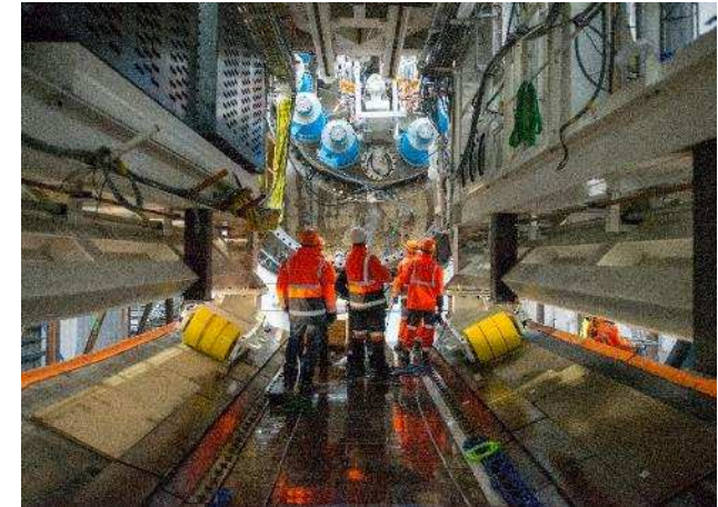
TBM (extension of Line 14 – Grand Paris Rapid transport project)
