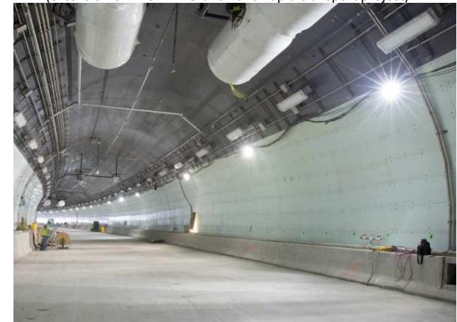
Port of Miami Tunnel – United States
