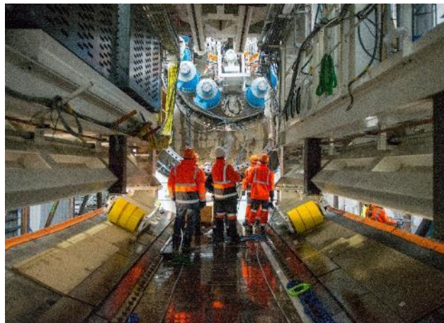
Tunnelier (prolongement L14 – Grand Paris Express)
