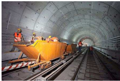
Metro line 3 – Cairo, Egypt
