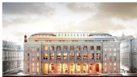
Conversion of Louvre post office into a mixed-use development – Paris, France
