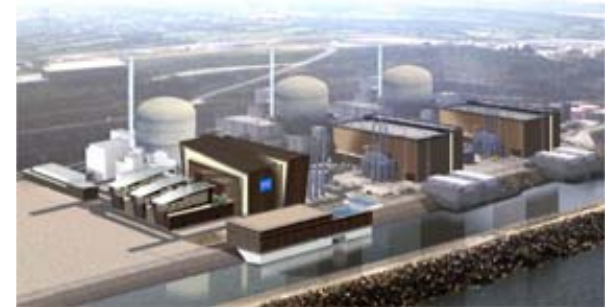
Flamanville site France
