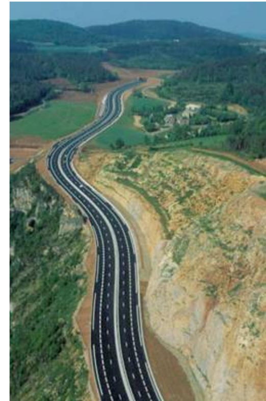
A75 motorway, France
