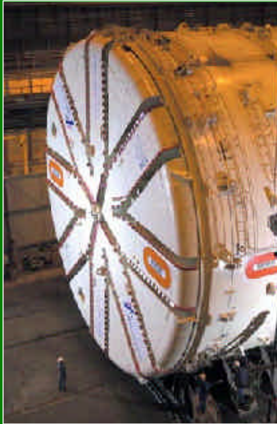
Groene Hart tunnel (Netherlands) €380m
