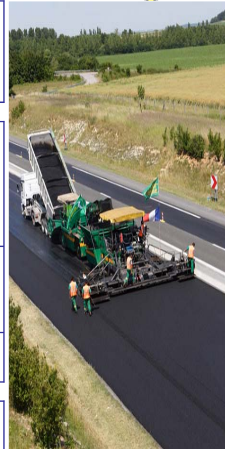
Autoroute A26 France
