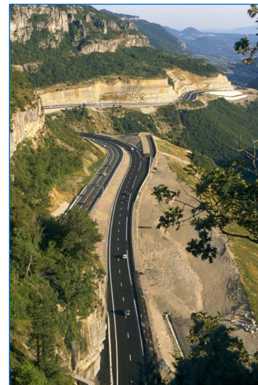
Autoroute A75, Hérault, France
