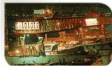
Kwun Tong bridge, Hong Kong
